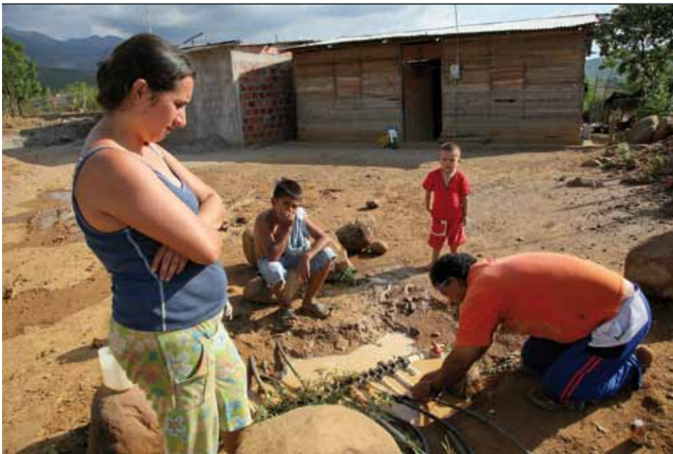
An IDP repairs a water pipe in the city of Cucuta, Colombia. Most IDPs who live in this poor neighbourhood are not assisted by any official bodies. (Photo: UNHCR/ Boris Heger, June 2010)
